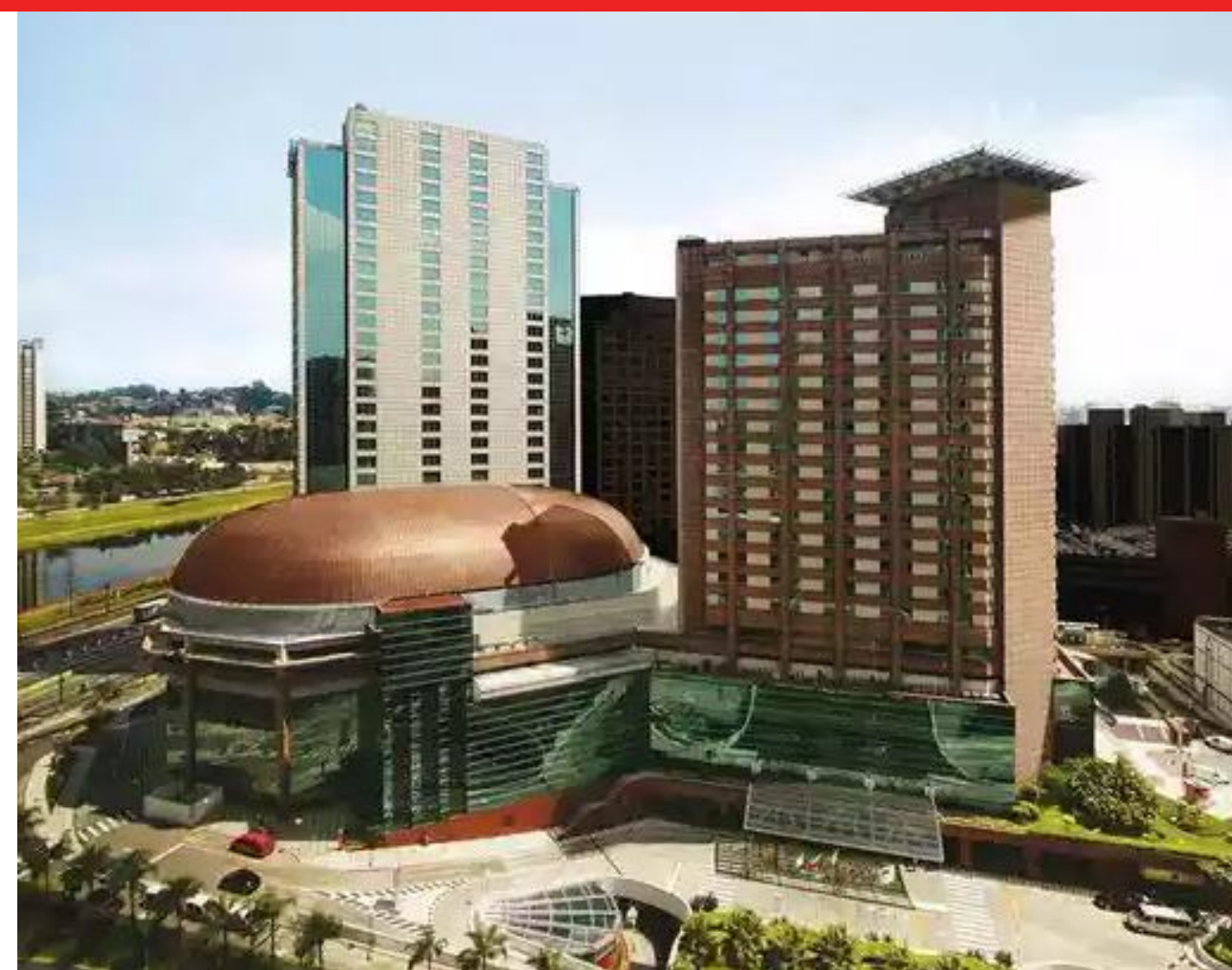
HOTEL SHERATON WTC AND WTC CONVENTION CENTER
